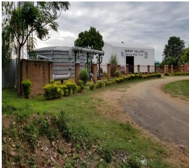
Karonga Water Supply Treatment Plant
